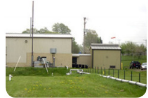
Groundwater Treatment Building
